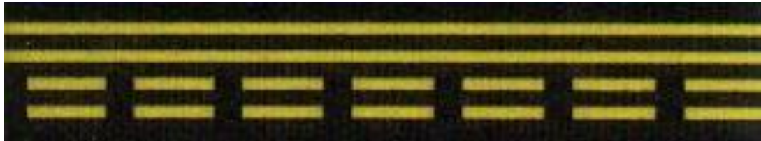
Runway Holding Position Marking
