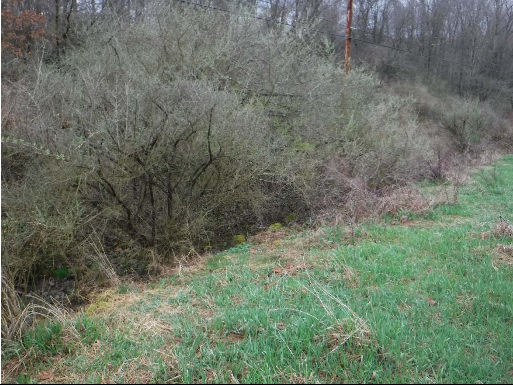
Photograph #5 | Vegetated and riprap lined drainage swale, southeastern perimeter of site
