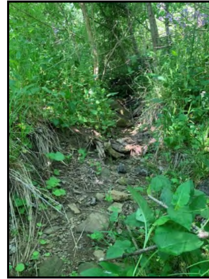
26) 05/25/2021: AGC Airfield north of runway 28, facing west and upstream in Channel 10. Channel 10 did not contain flowing water.
