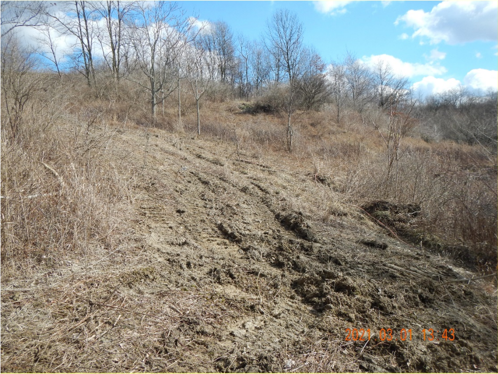
Photograph 4. Looking south at dozer clearing near Boring B-7.
