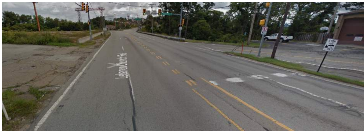
Existing Driveway Location Opposite Rodeo Dr East
