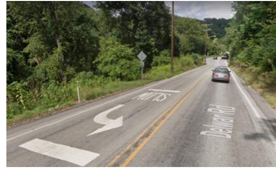
Northbound towards SR 2046 (Streets Run Rd)
