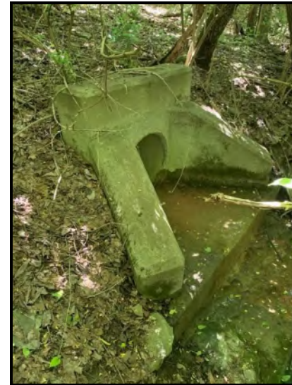
24) 05/25/2021: AGC Airfield west of runway 10, facing south at the outfall upstream of Channel 9.
