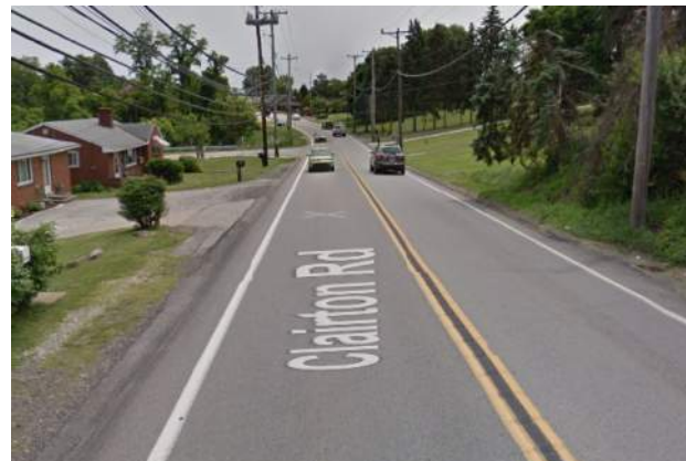
Southbound South of Lebanon Church Rd
