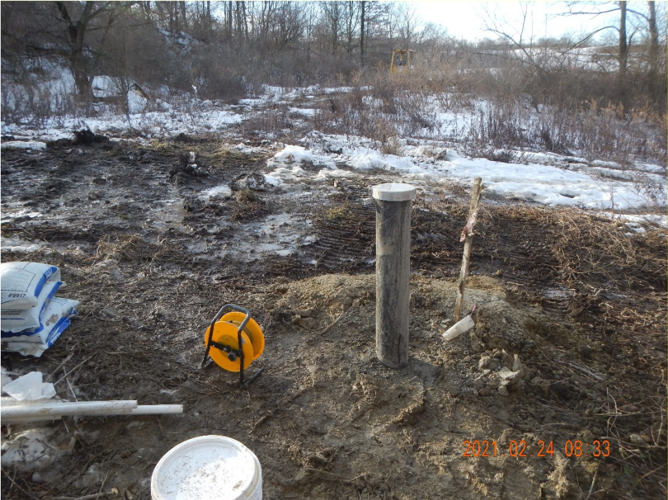
Photograph 2. Looking south at monitoring well installation at Boring B-5.
