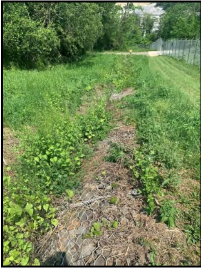
29) 05/25/2021: AGC Airfield east of runway 28, facing north and downstream of Channel 12
