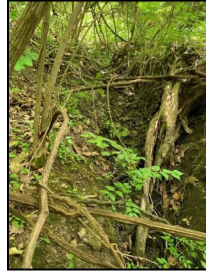
22) 05/20/2021: AGC Airfield west of runway 10, facing northeast and upstream in Channel 8.
