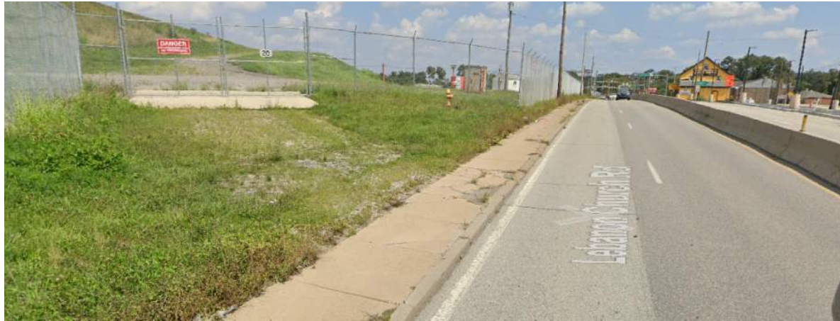
Existing Airfield Driveway Location Opposite Rodeo Drive West
