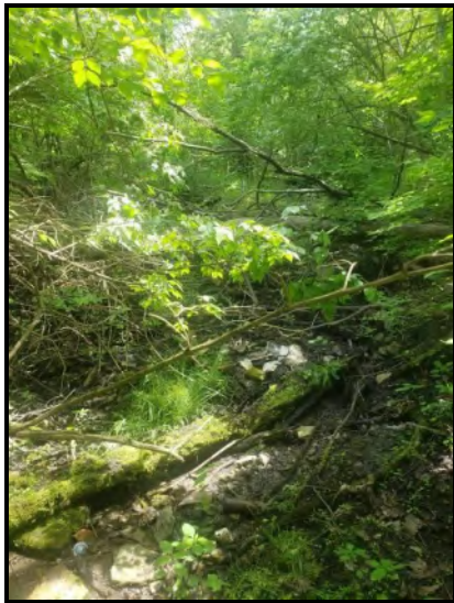
15) 05/20/2021: AGC Airport west of runway 10, facing west and upstream in Channel 5.
