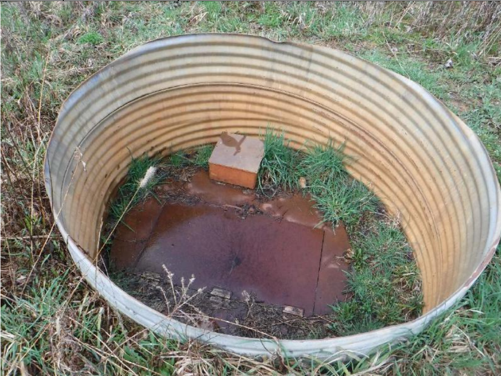
Photograph #22 | Leachate sump, southern portion of site
