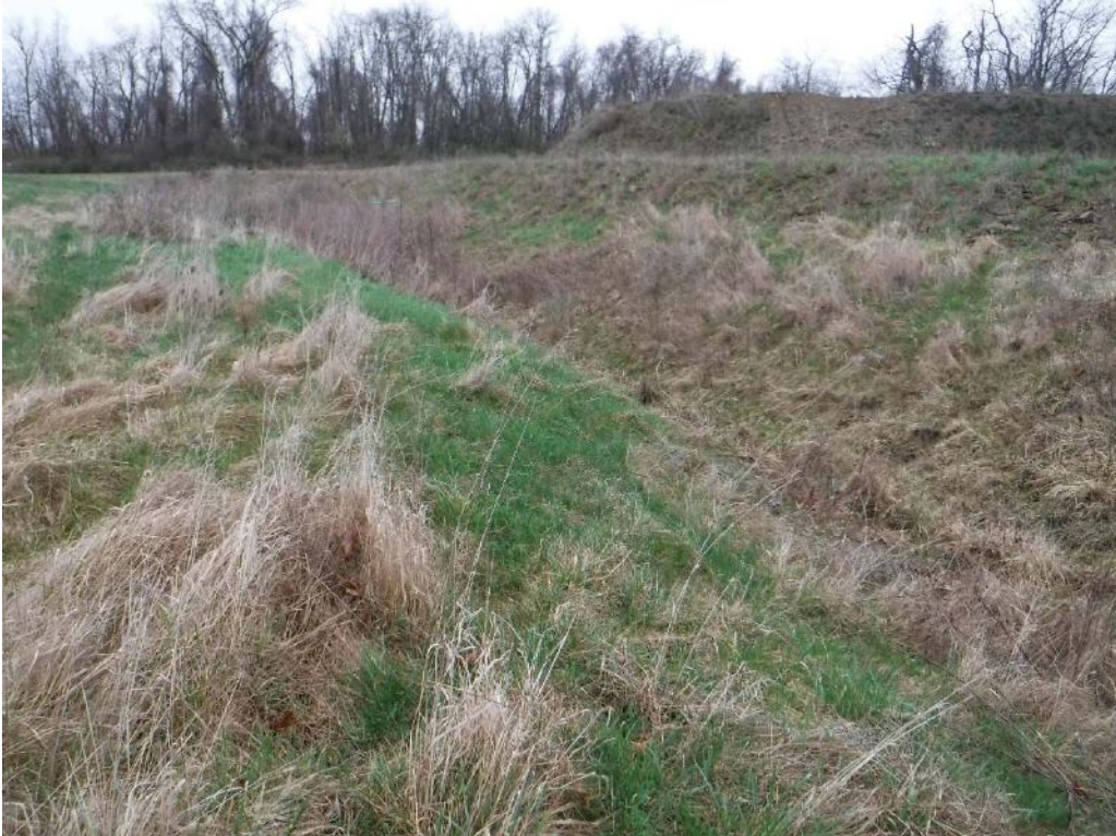
Photograph #4 | Drainage swale, northeastern perimeter of the site
