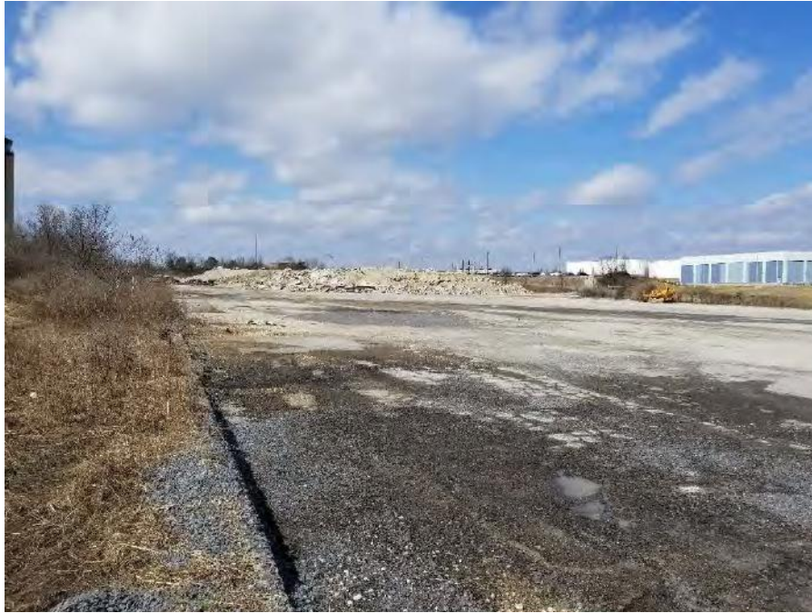
Photograph 1: West view of southwest portion of AOI.
