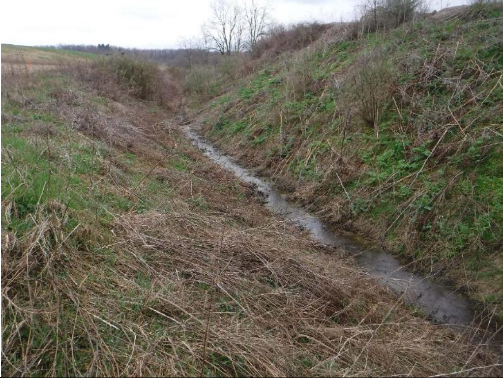
Photograph #3 | Drainage swale, northern perimeter of the site
