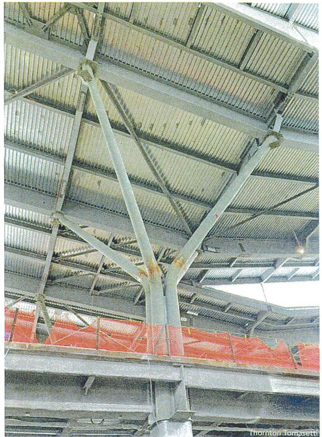
below: The tree columns are spaced as far as 120 ft apart.
